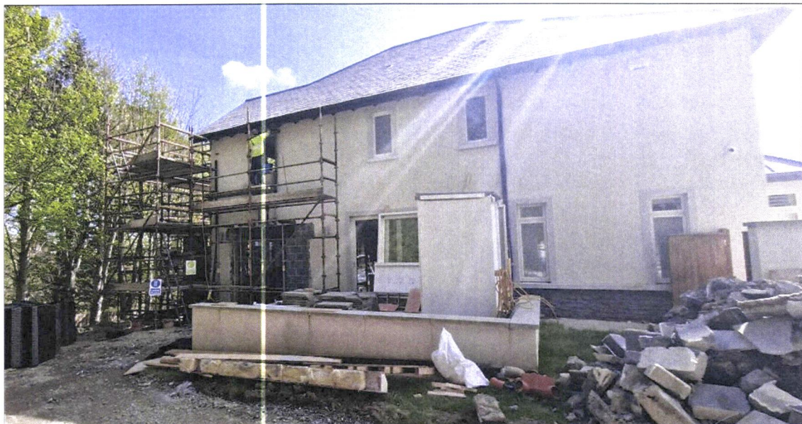
Figure A2: Rear Elevation, Under Construction, Showing Inclusion of Window
