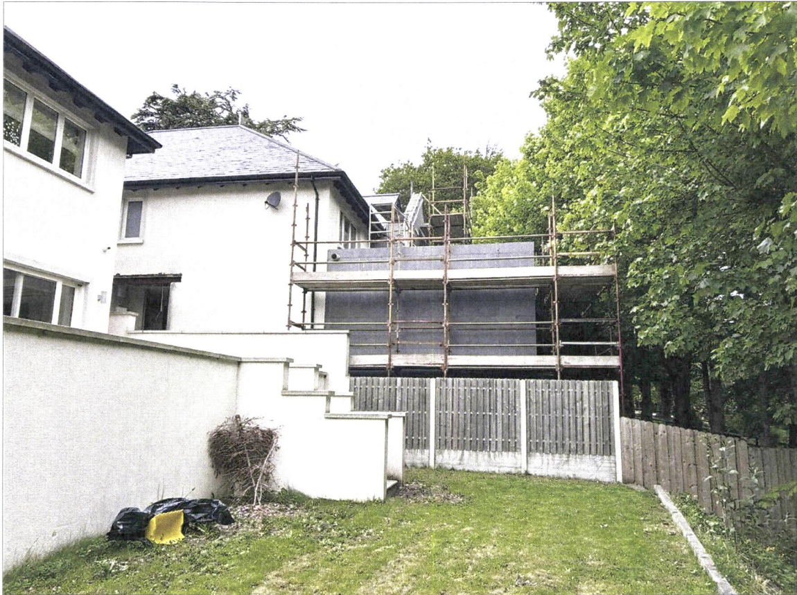
Figure A3: Rear Elevation, Under Construction 01.06.2026
